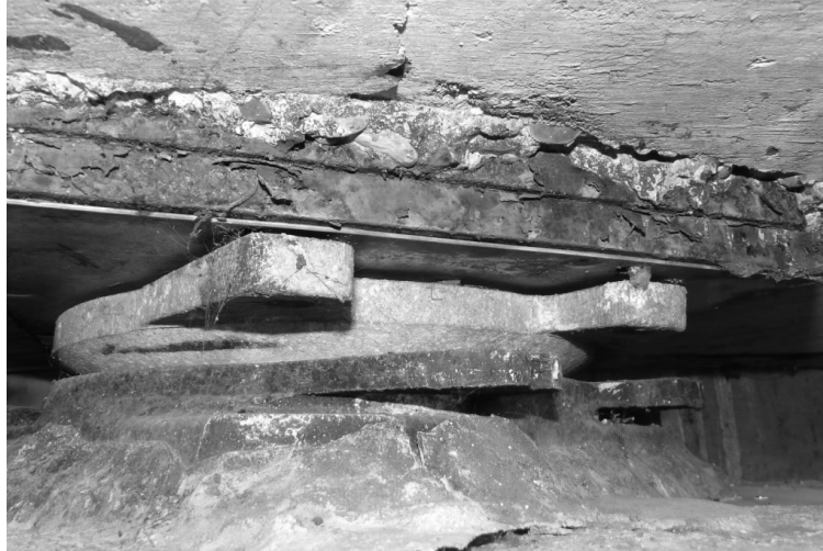
Vicarage bridge bearing
